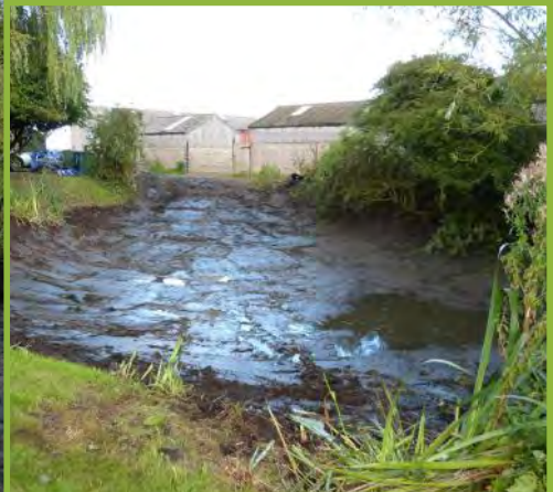
Empty, after removal of reeds and dredging of silt
